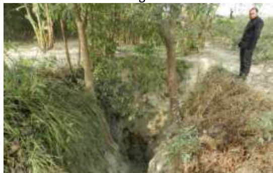
Motors are installed 3-4m below ground to draw water from irrigation borewells
