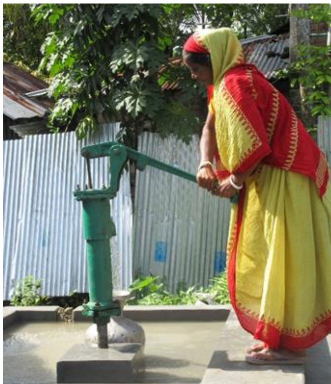
A new DTW, green means: "no arsenic"
