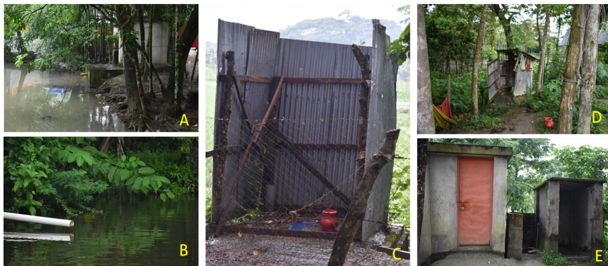
Figure 12: Existing WASH infrastructure in Vedurua and Dhanua Union in Bhola Sadar (A)(B) Mouth of the toilet outlet placed directly over the wetland. (C)(D)(E) Toilets having no proper sewage disposal mechanism in Vedurua and Dhanua Union in Bhola Sadar.
